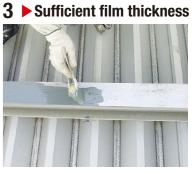
Apply two coats. (Each coat: 40µm) Total dry film thickness = more than 80µm Do not spread the paint too thin. Anti-corrosion performance is proportional to dry film thickness. Coating interval : 30~60min
